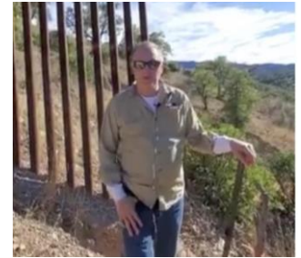
Above: Congressman Biggs standing between the end of the border fence structure and the 4-strand barbed wire fence that marks the international boundary
