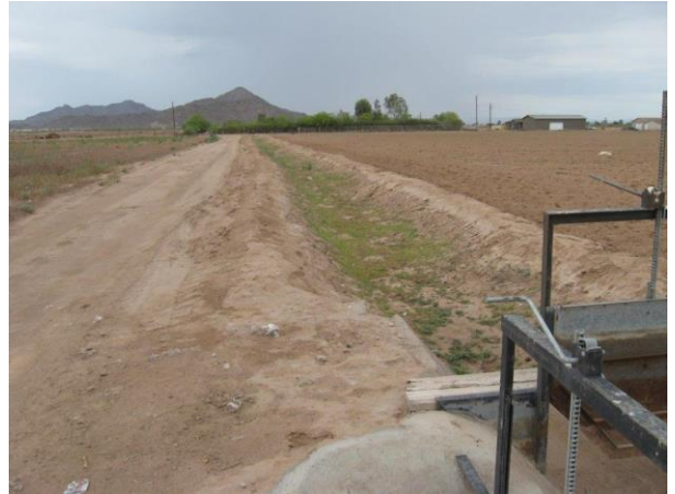
Above: unlined water ditch
