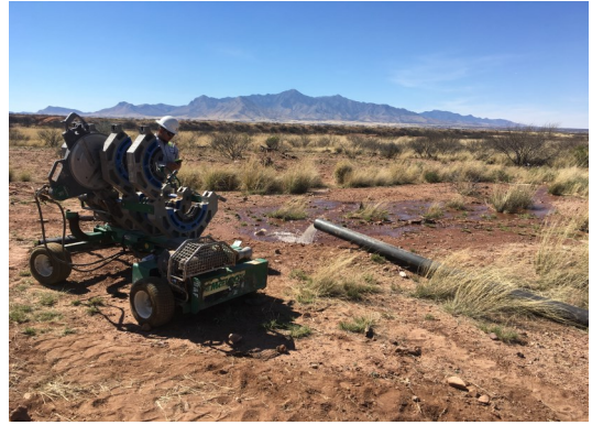
3/17/17 Water Line Completed
