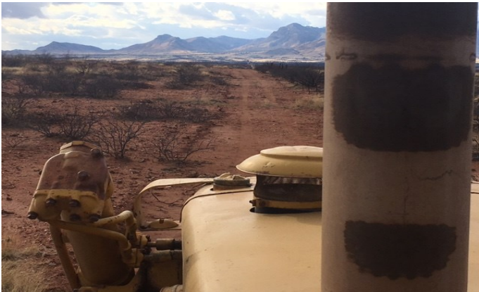
2/15/17 Road improvement to site
