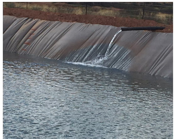
3/28/17 Filling water pond
