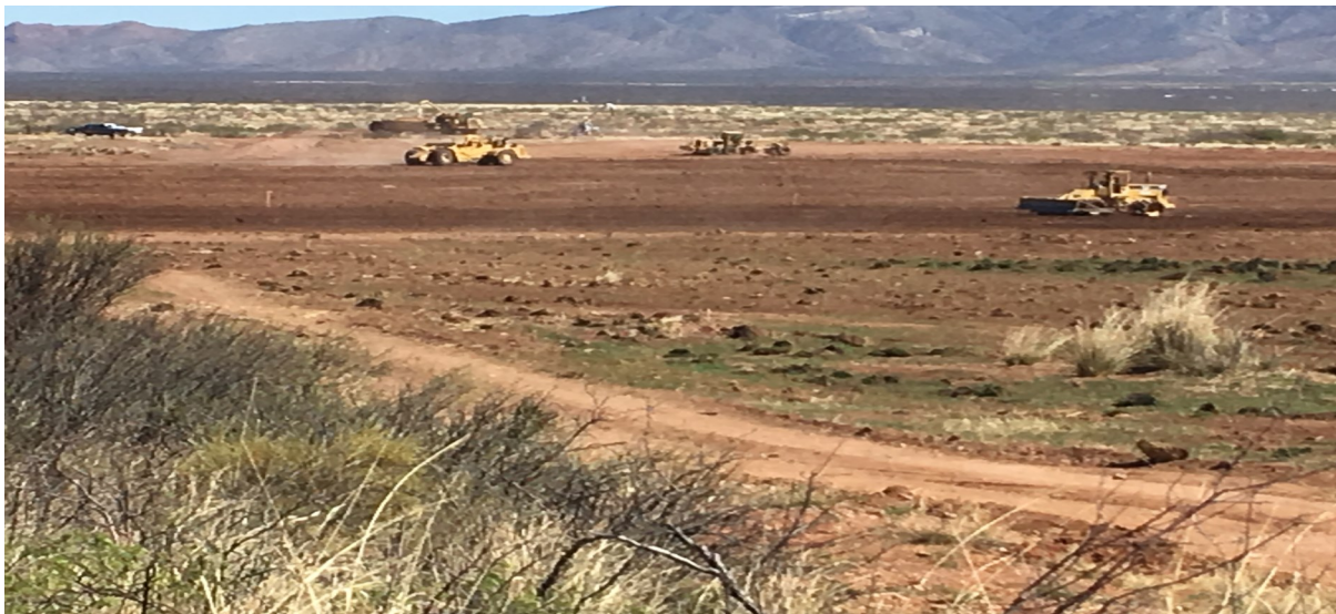
3/30/17 Detention basin earthmoving
